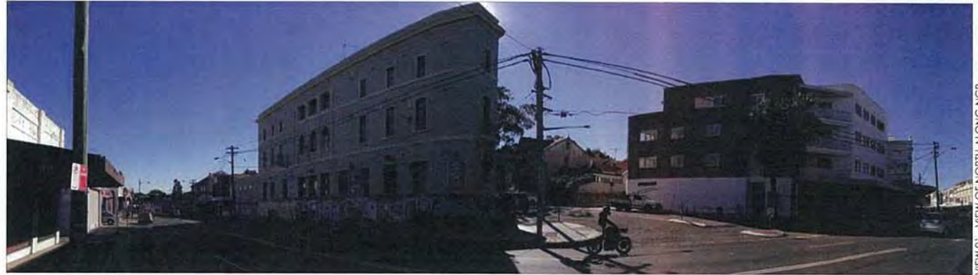
VIEW 01 - VIEW OF NORTH ALONG NCR
